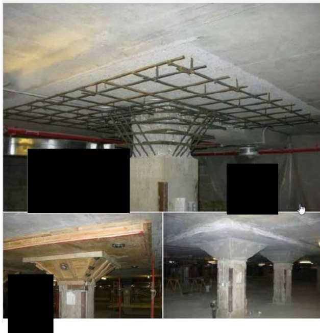
Figure 5.1 Shear collar for columns
